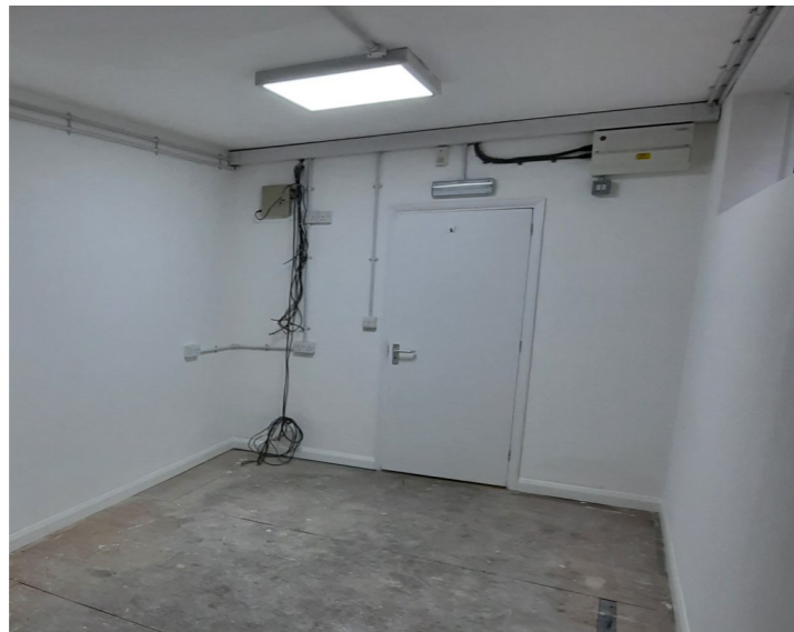
Kitchenette & WC Area
